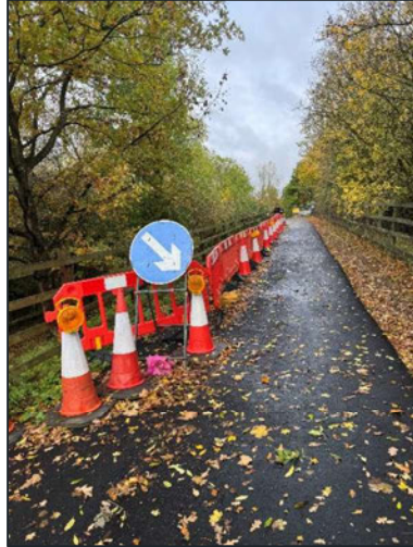
M11 Overbridge Approach
