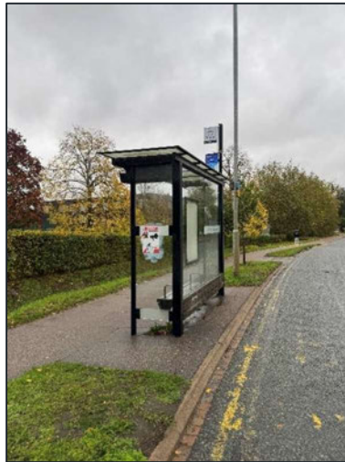
Sheltered Bus Stop
