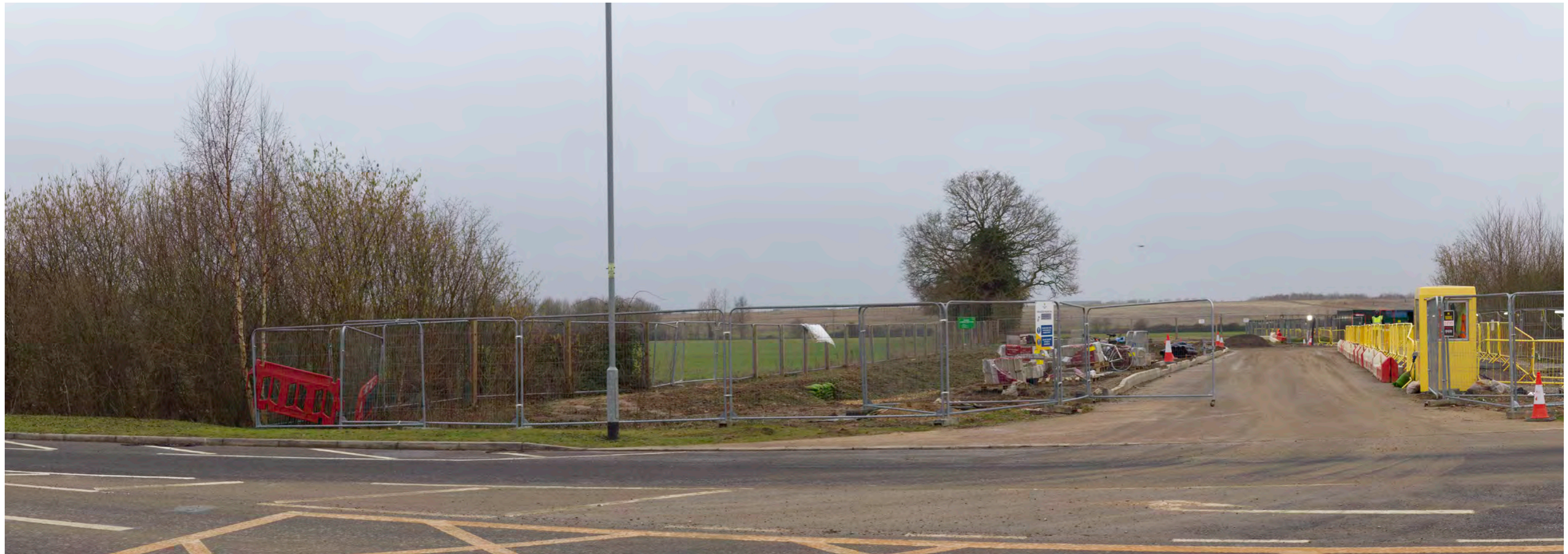
Representative Viewpoint 2 (Left-centre) - Entrance to Milton Park and Ride
