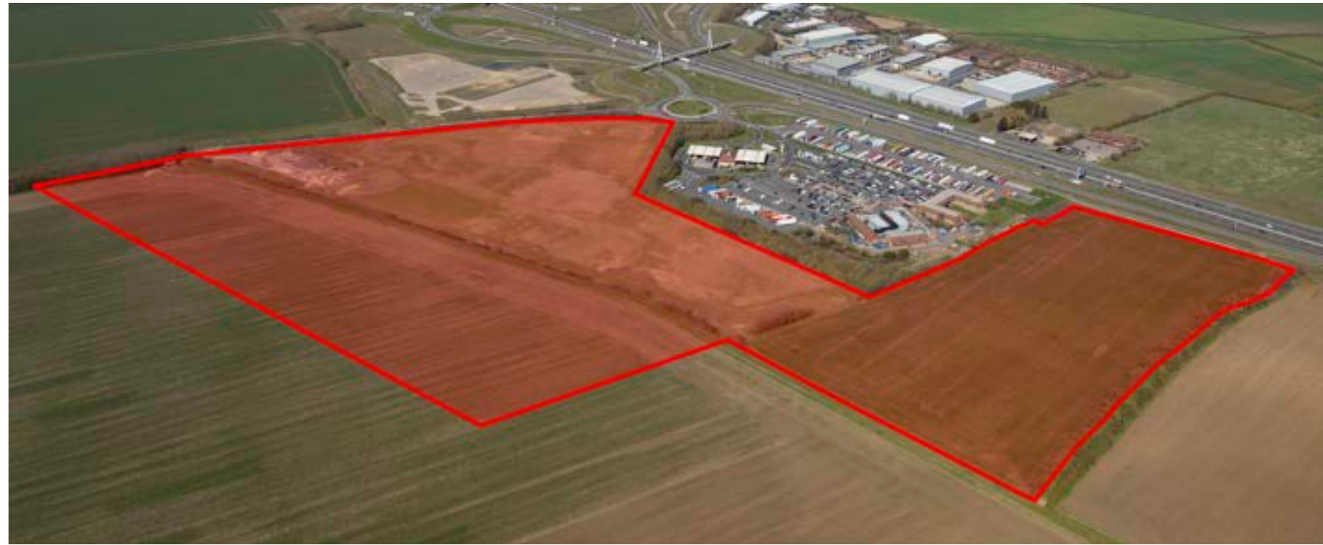
Figure 3: Aerial view of the Site looking north-west
