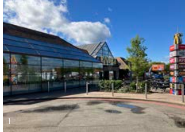
Figure 6: Cambridge Services Facade
