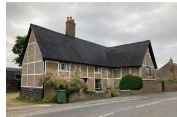
Grade II Listed - 279, High Street
