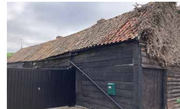
Examples of the original agricultural buildings in weatherboarding. Some with clay tiles (pictured) or metal corrugated roofs.
