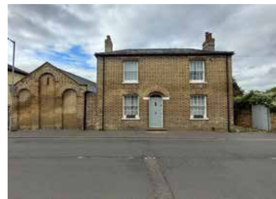
Grade II Listed - 86, High Street
