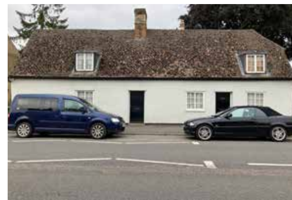
Grade II Listed - 226 & 228, High Street
