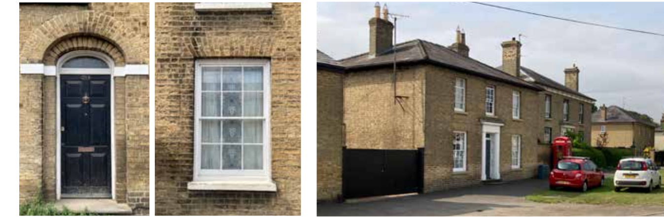
Brick detailing over doors and timber sash windows is a common architectural features found in the village on both larger villa properties and former worker cottages.
