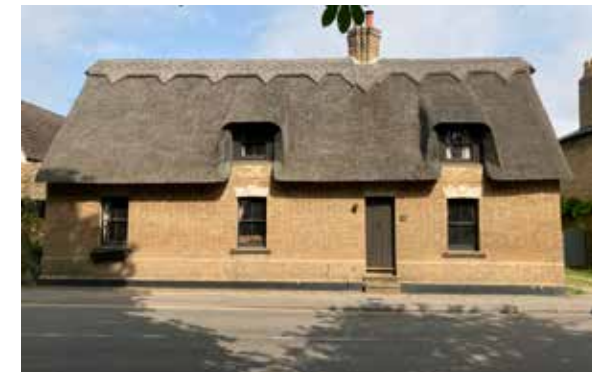
Grade II Listed - 332, High Street
