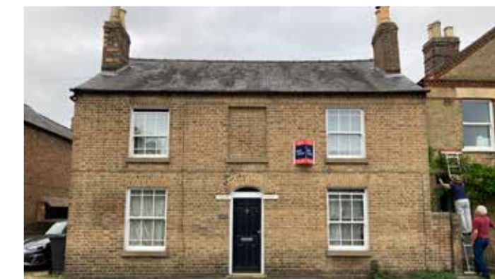
The local buff brick with a slate roof covering is the predominant material found on buildings within the village.
