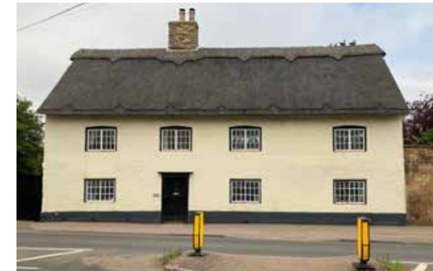
Painted brickwork is also found on a number of buildings within the village.
