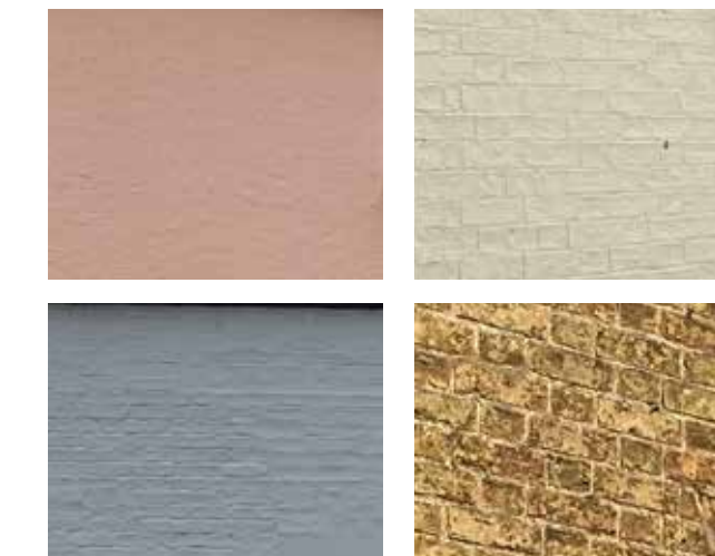
Examples of the subtle and muted colour palette found on the more historic buildings around the Cottenham.
