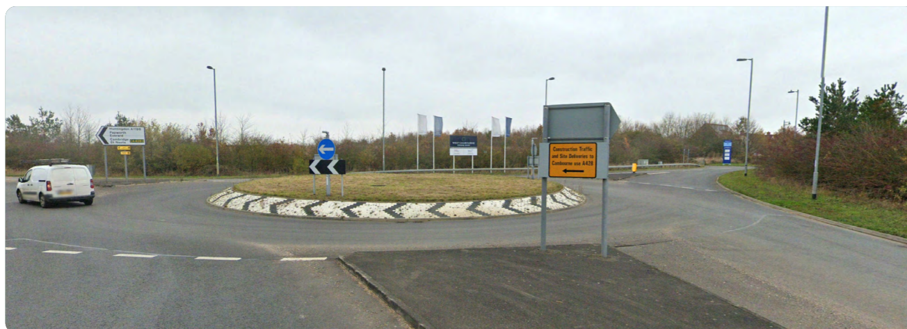
▲ Existing School Lane roundabout
