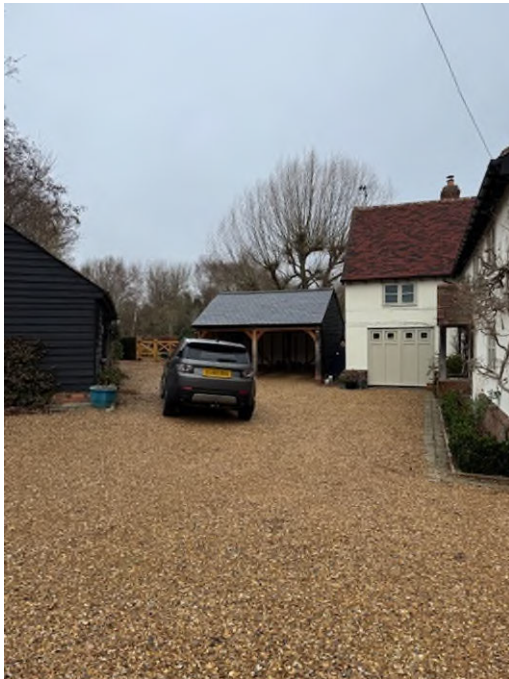
View of Swans Corner to North showing part residential dwelling, ancillary residential and car parking within the Green Belt
