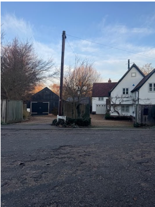
View North showing crossover and gate already formed onto 'self build' plot and separate adjacent crossover and gate to Swans Corner.
