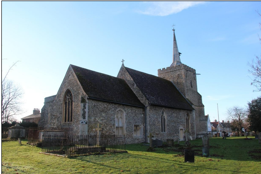
Figure 2.6 Parish Church of St Mary and St John the Evangelist (top) and example view to the Church from the Site looking south-west (bottom)
