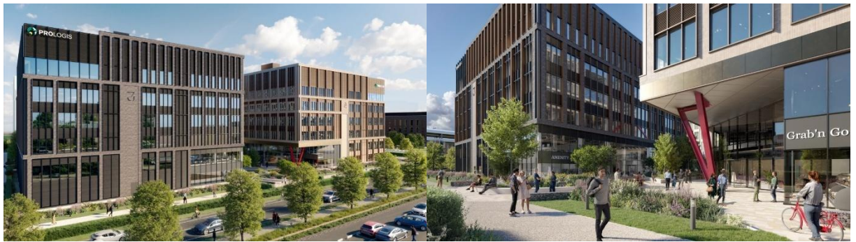
Figure 11 - Building 2000 Discovery Place - City Centre Periphery Office Under Construction
