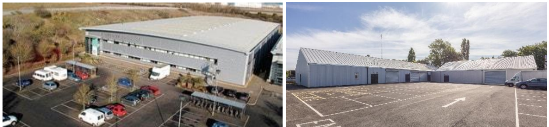
Figure 31 - Unit 9 Norman Way & Unit 8 Coldhams Road – Available & Existing Industrial / Light Industrial Space – City Core
