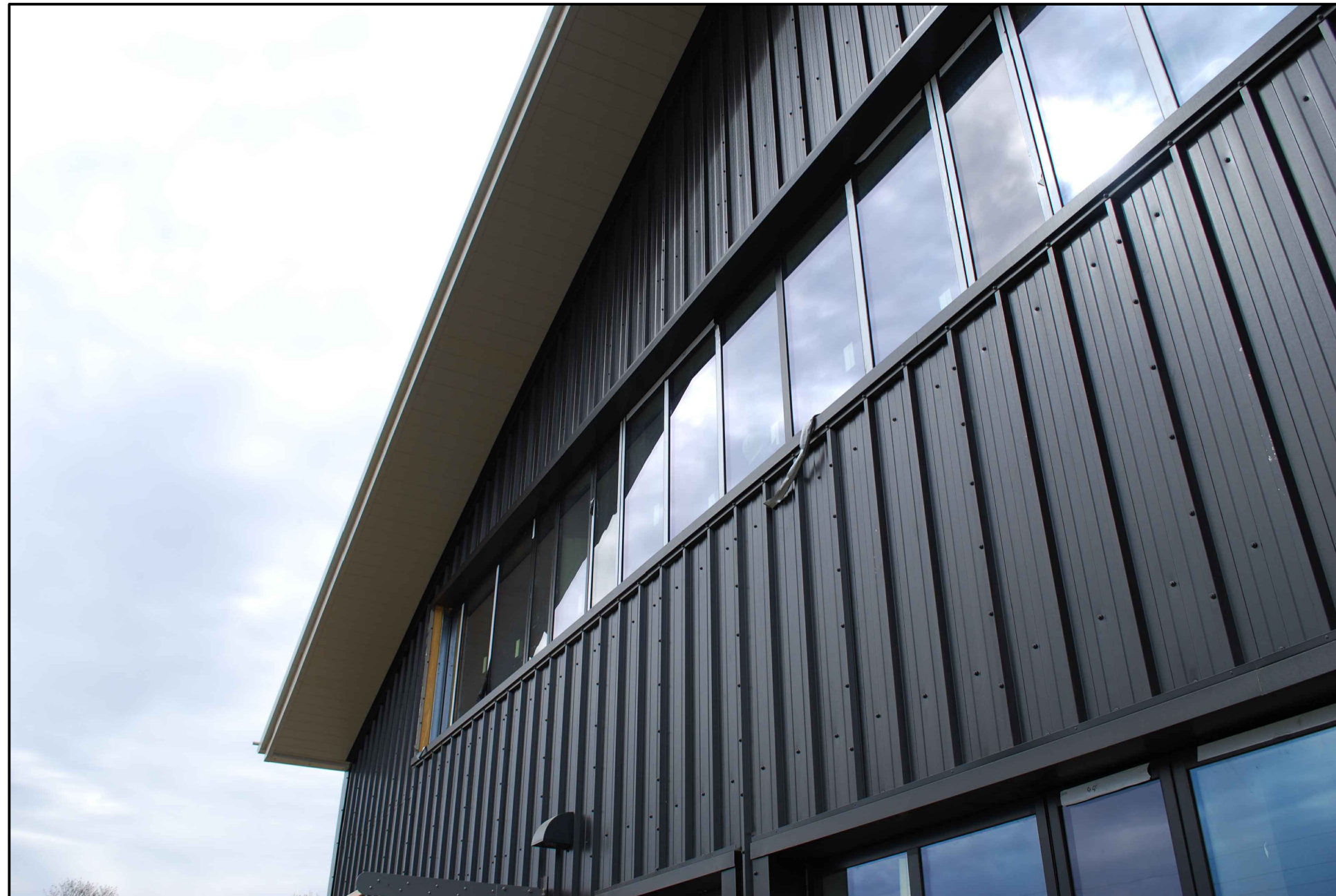
Examples of windows within cladding and full height glazing to pitched elevation
