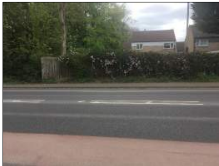
Photograph 2: Pedestrian Footway on Bridge Road
