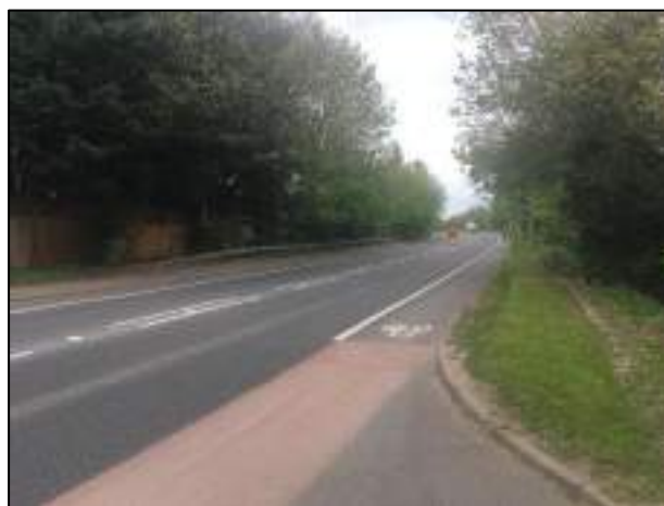
Photograph 1: Bridge Road Conditions
