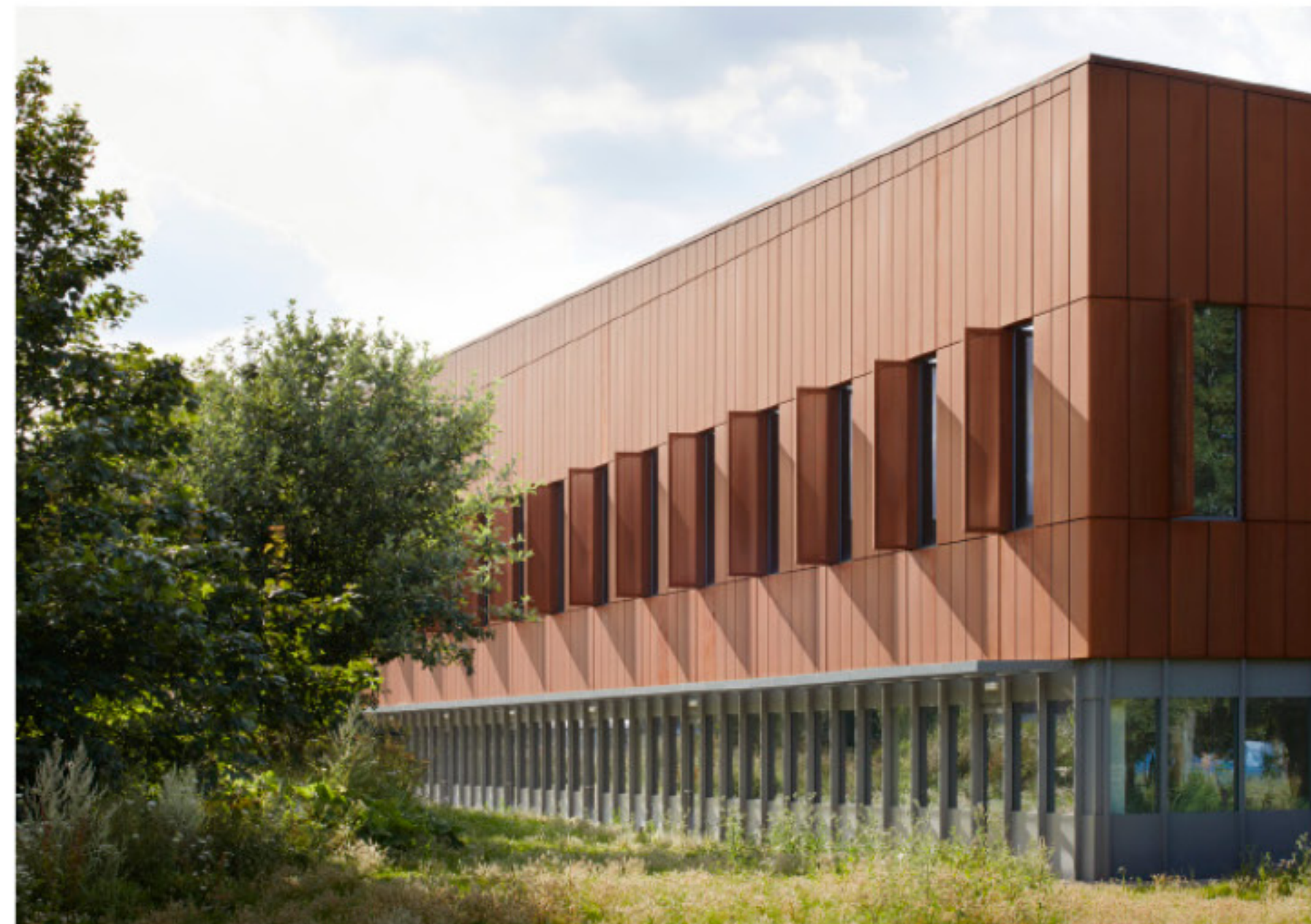
Mid-tech building, Harwell Oxford, Allies and Morrison
