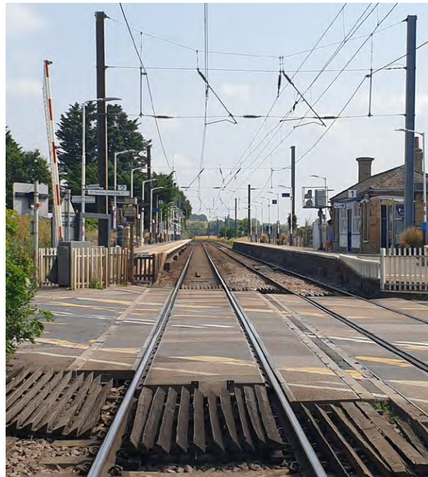
A10 Foxton level crossing
