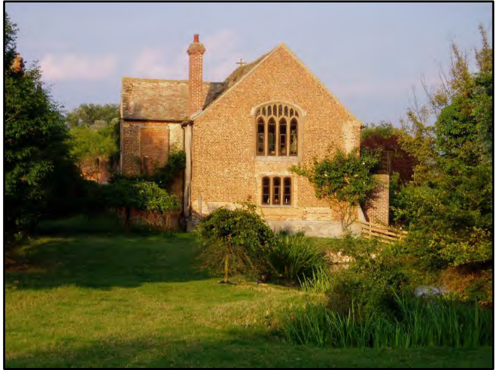
Plate 2: Chapel to the South West of Childerley Hall (Wikimedia Commons, 2005)
