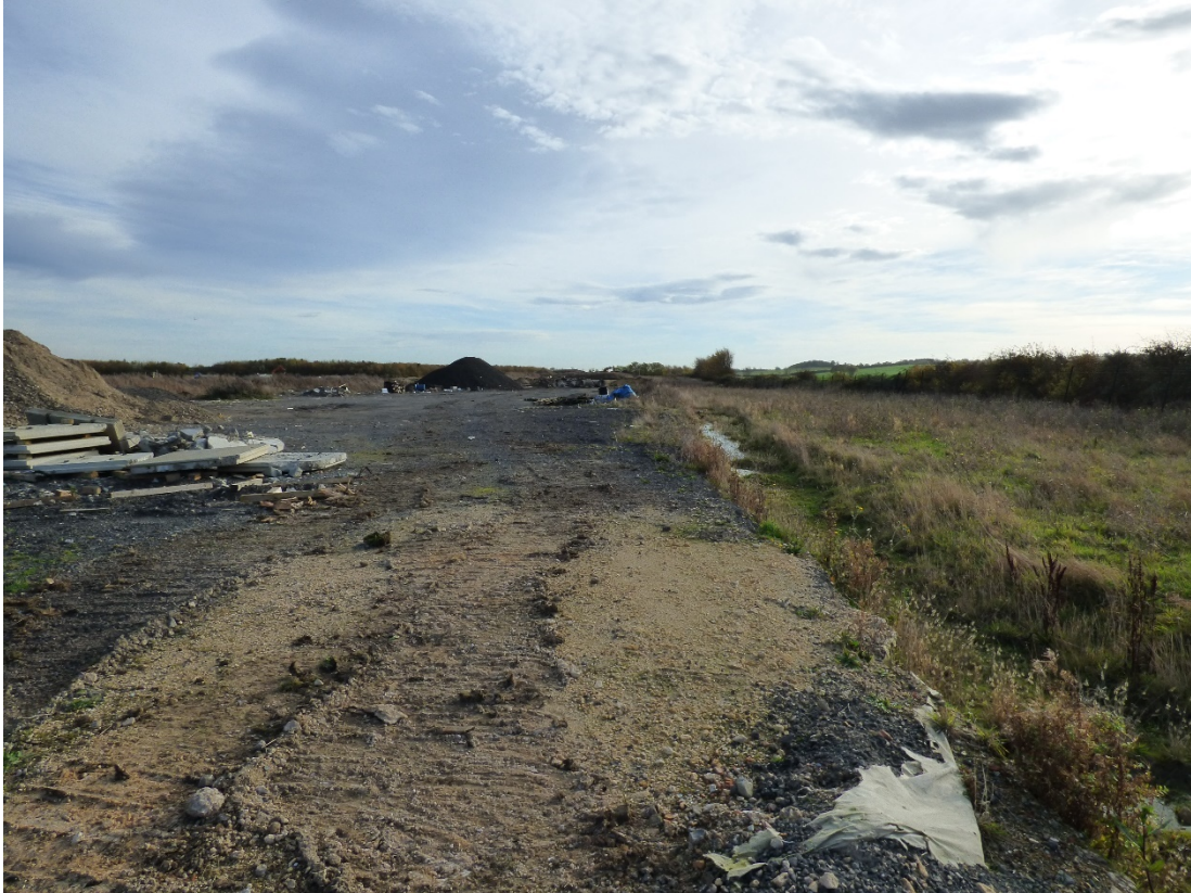
View looking south-east along the southern boundary Fig 11
