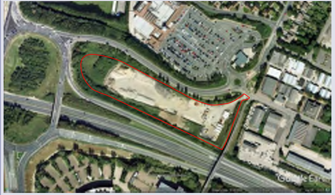
2006: onsite: the majority of the site is in use, potentially as a temporary works area associated with road/junction improvements which are in construction to the NW side of junction 33 on the A10. Several stockpiles are shown across the central and western parts of the site. Additional storage/temporary buildings are also shown in the east (October 2006)
