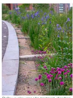
Shallow swales using edge treatment, absorbing energy from runoff
