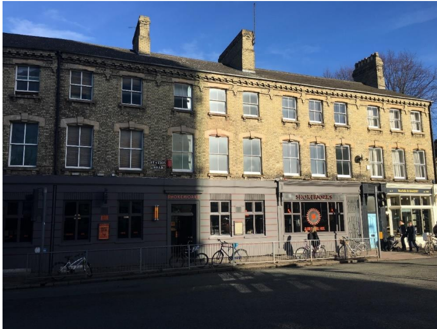
Figure 18: view of 5 - 7 Hills Road
