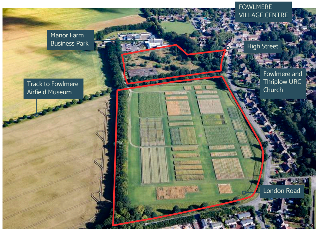
View looking north across the site with Fowlmere village centre in the background
