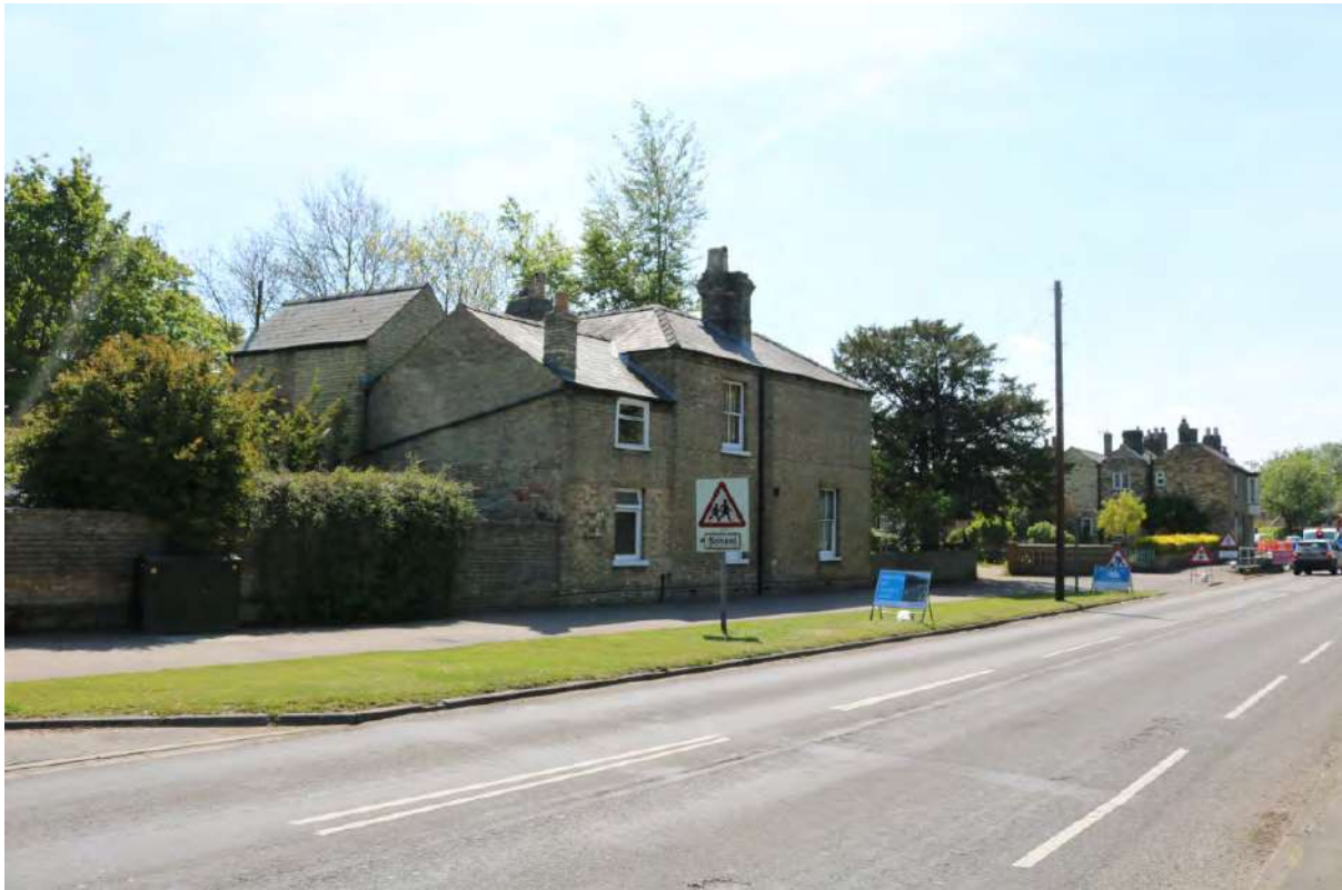
Image EDP 1: View east along Glebe Way.
