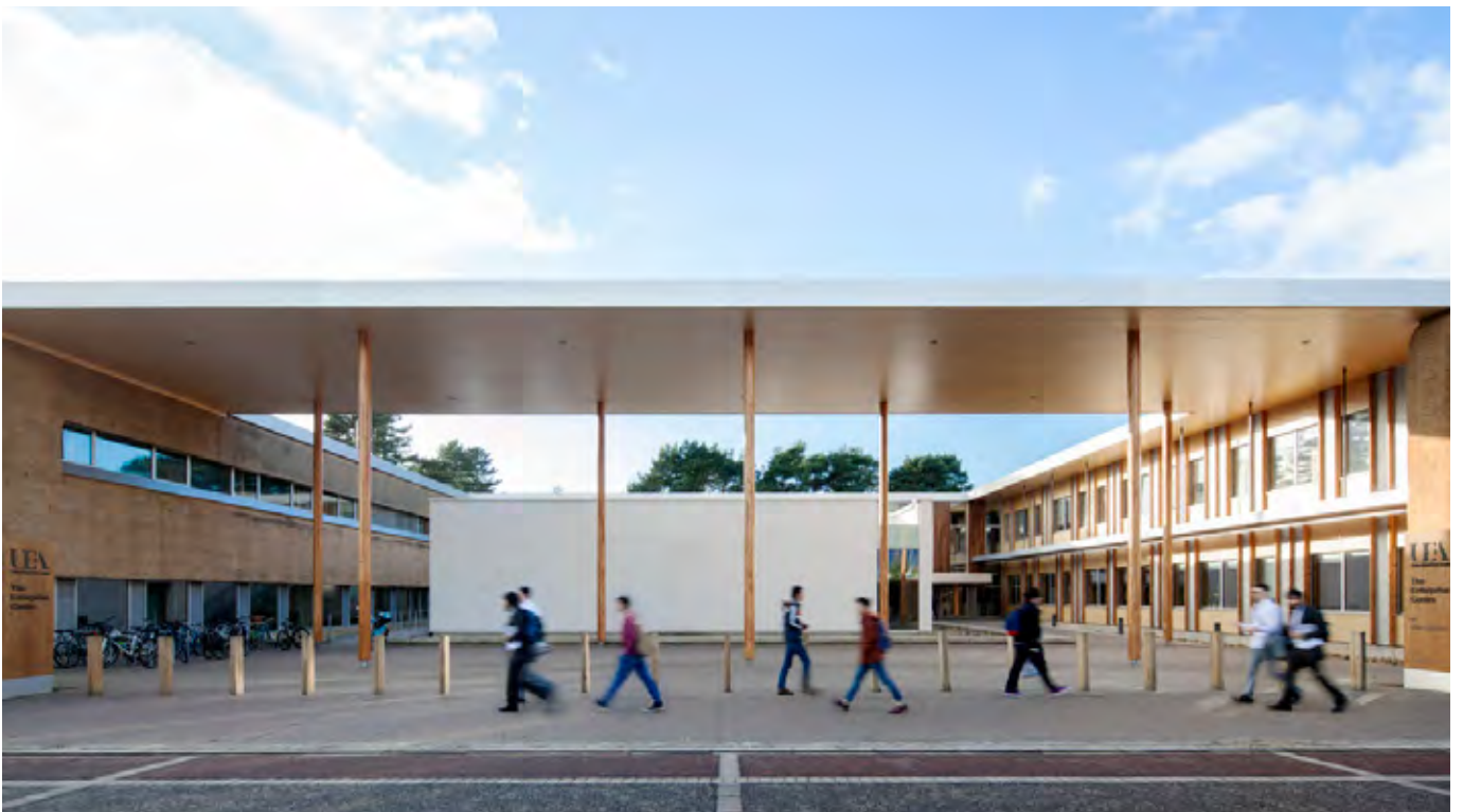
Figure 36 - Enterprise Centre University of East Anglia, Norwich. Net Zero Carbon University building built for no extra cost.
