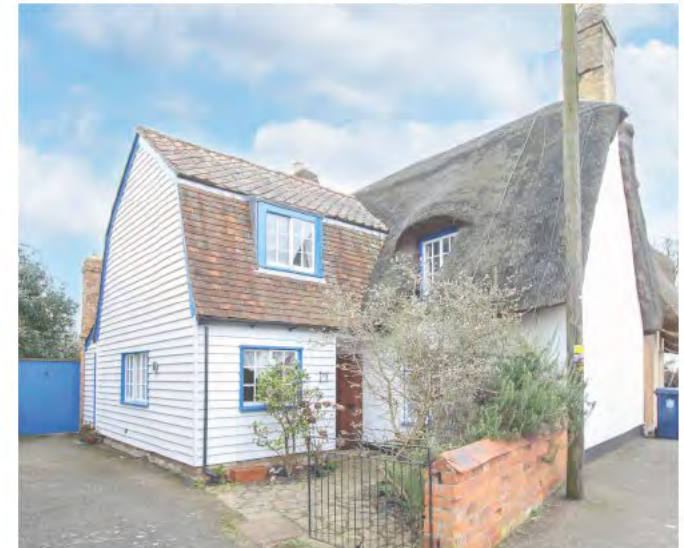
Figure 25: Thatched roof house with white cladding
