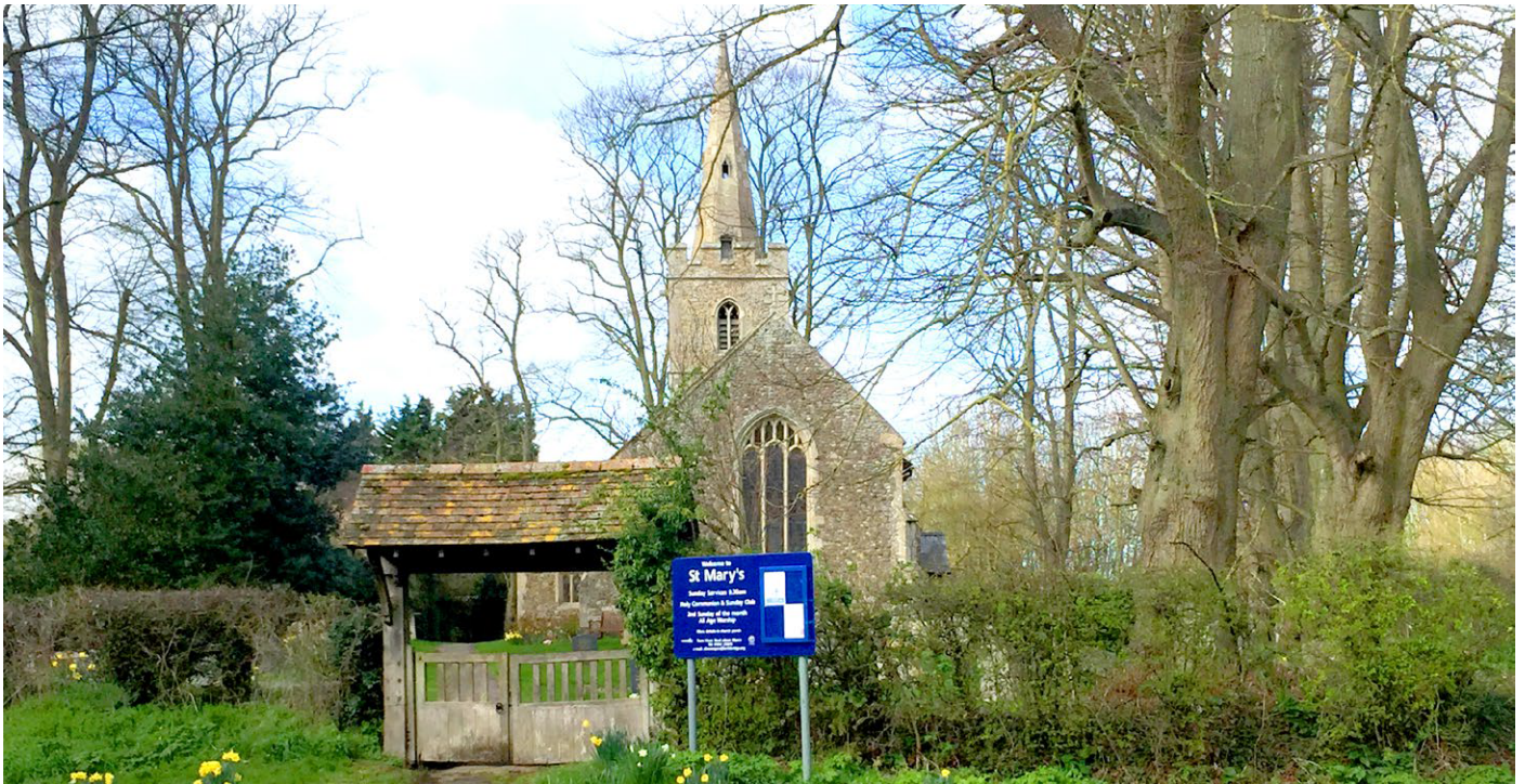
Parish Church of St Mary (Grade II* Listed)
