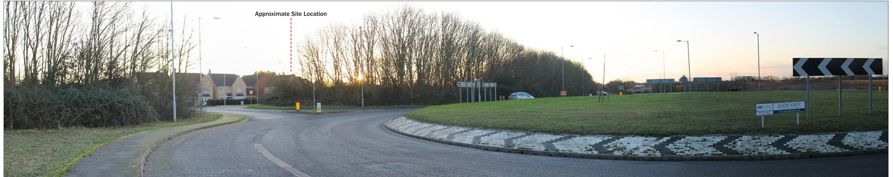
Photo Location 13: View looking south west towards the Site from St Neots Road / A428 roundabout.
