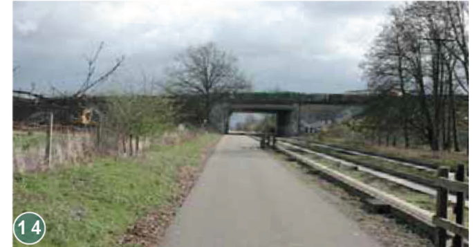
Figure 30; The Guided Busway crossing the A14
