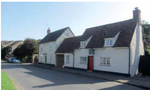
Figure 14 Photographs Exemplar and Reference Buildings Cottages Steeple Morden
