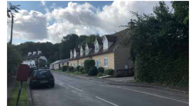
Reference building (development at Madingley)
