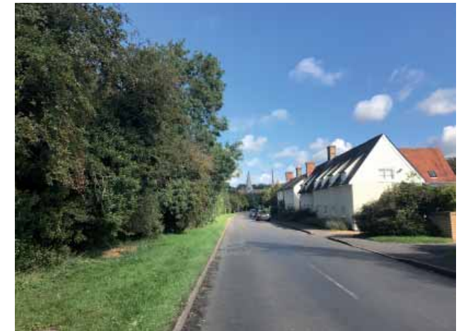
Figure 2 Photos of context Cottages Station Road (Conservation Area)
