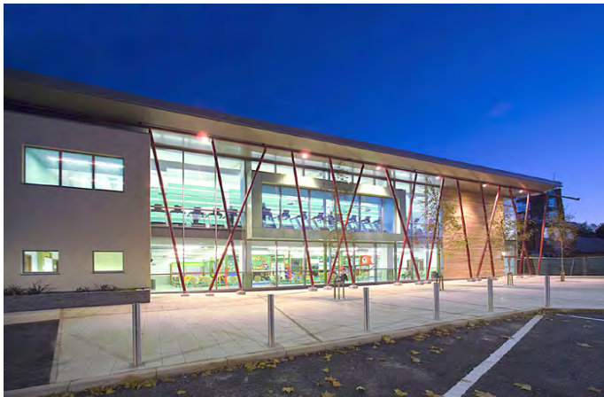
MULTIPURPOSE HALL AND GYM
