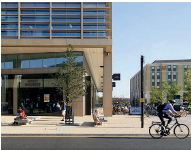
Station Square has transformed the arrival experience in Cambridge
