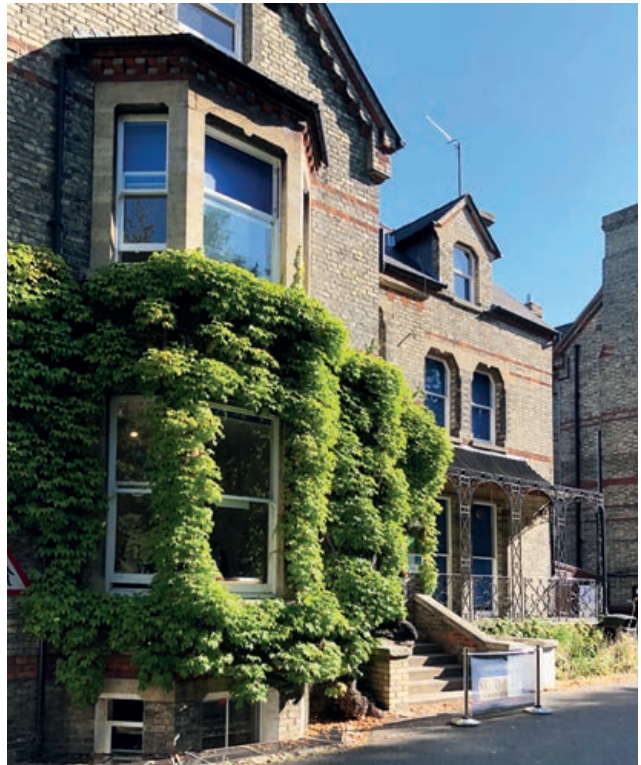
Front of 6 Salisbury Villas; typical architectural qualities
