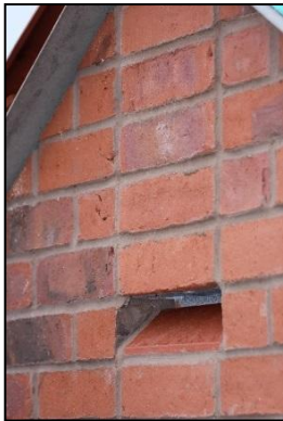
Figure 2: Habibat Bat Box faced with red brick, incorporated within wall at gable end
