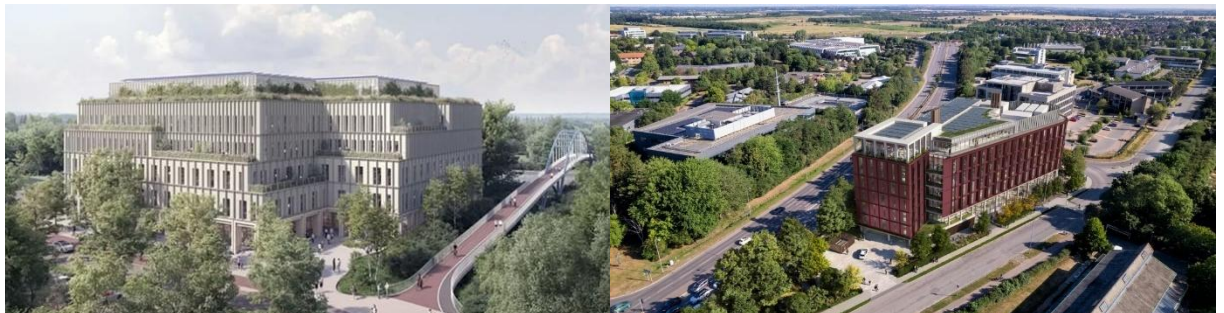
Figure 12 - Vitrum Building & Merlin Place - 'Northern Cluster' submarket Offices Under Construction
