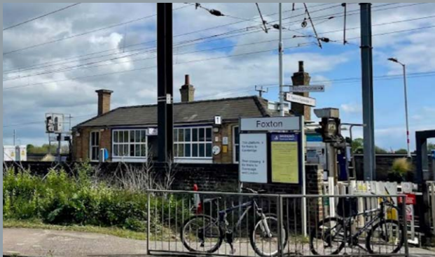
1. Foxton Train Station (source: Google)
