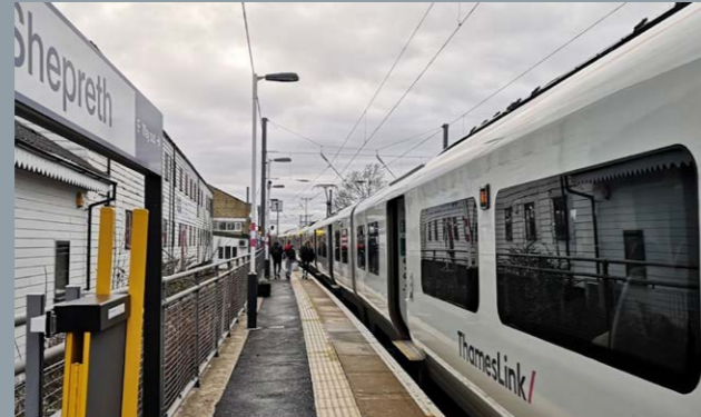
4. Shepreth Train Station (source: Google)
