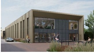
CGI of Phase 1 (Redevelopment strip out progressed)
