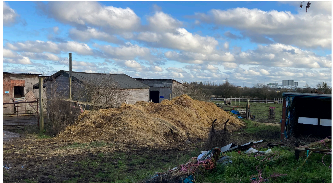
Figure 1; Cluster of agricultural buildings (equine facilities) within the site
