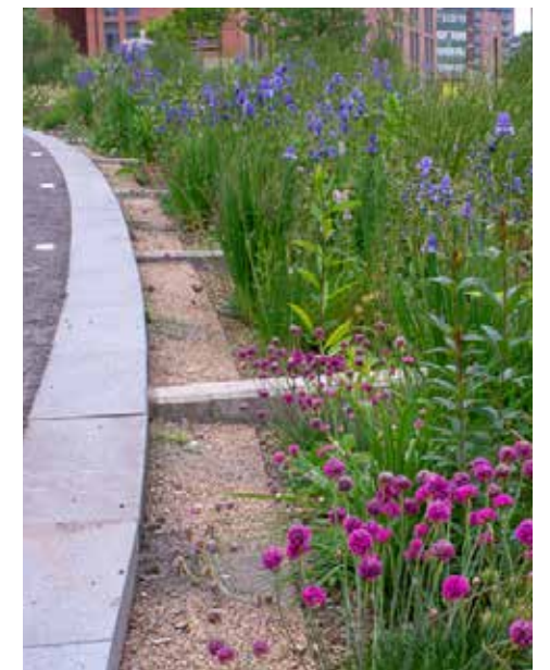
Shallow swales using edge treatment, absorbing energy from runoff
