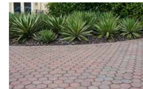
Permeable paving as a source control measure
