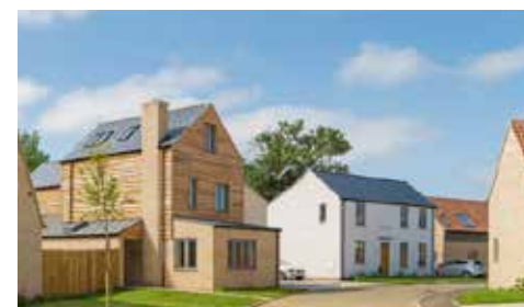
2 storeys and potentially loft occupancy
