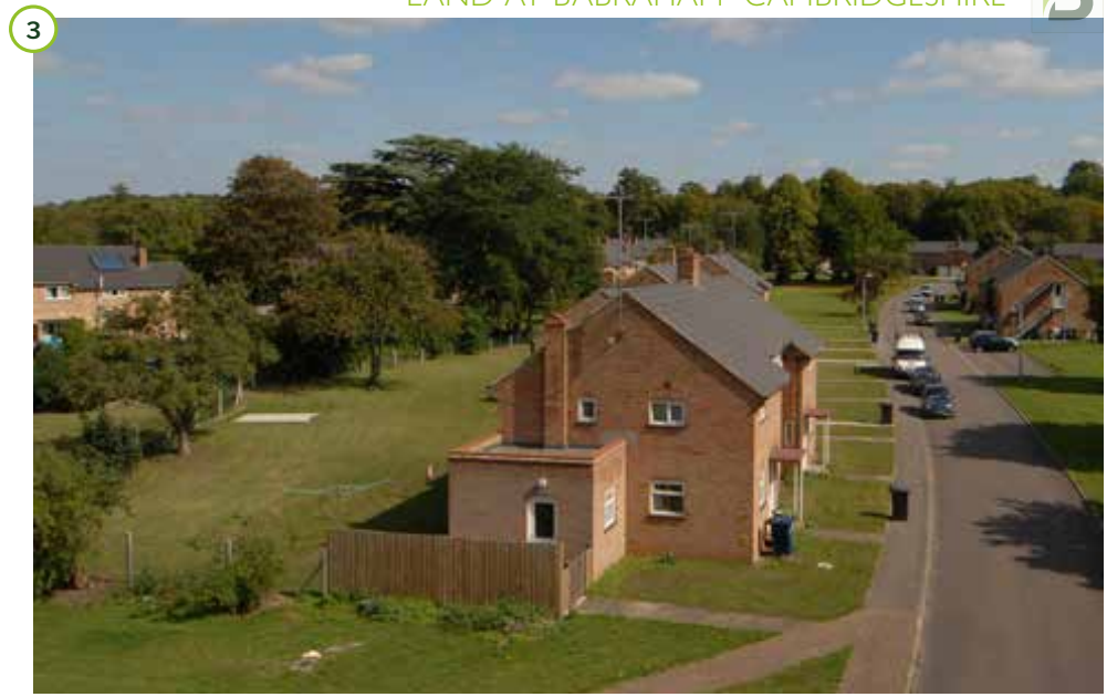
3 BRC accommodation, located north of the high street
