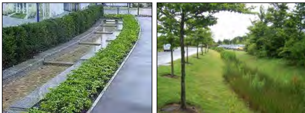
Figure 7.4: Open Swale / Rills Example
