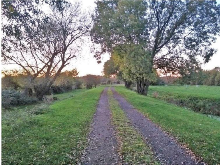
**Figure 3:** Much of the former rail alignment remains as an elevated embankment suitable for reinstatement (Photo: C. Ross 2019).
