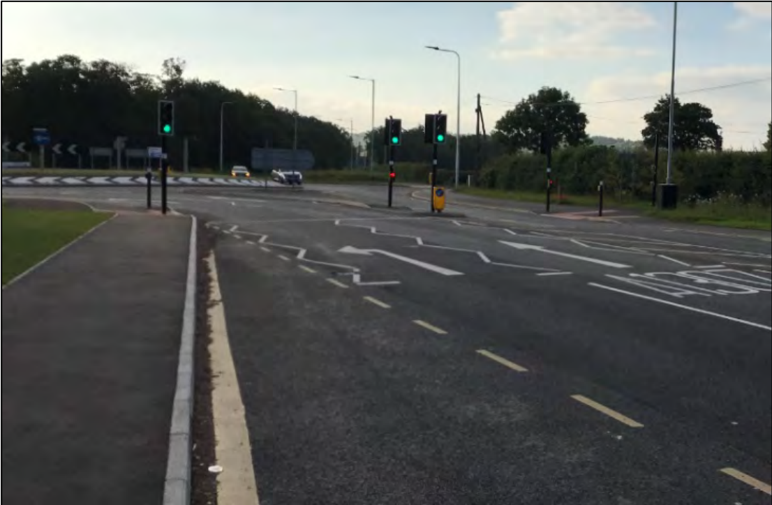
Figure 5: New Toucan Crossing on A1307 Immediately Southeast of Site Access Roundabout
