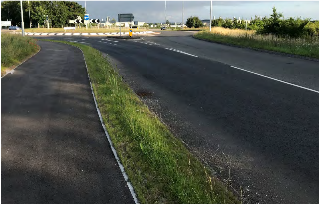
Figure 8: Photograph Showing Northwest Entry to A1307 Roundabout
