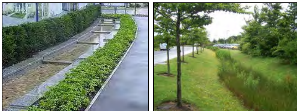
Figure 7.4: Open Swale / Rills Example
