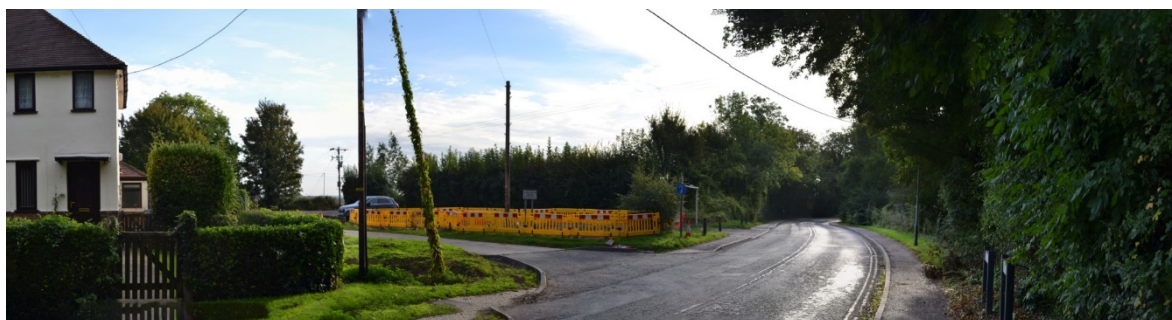
Figure 8: High Street/Teversham Road view from north
