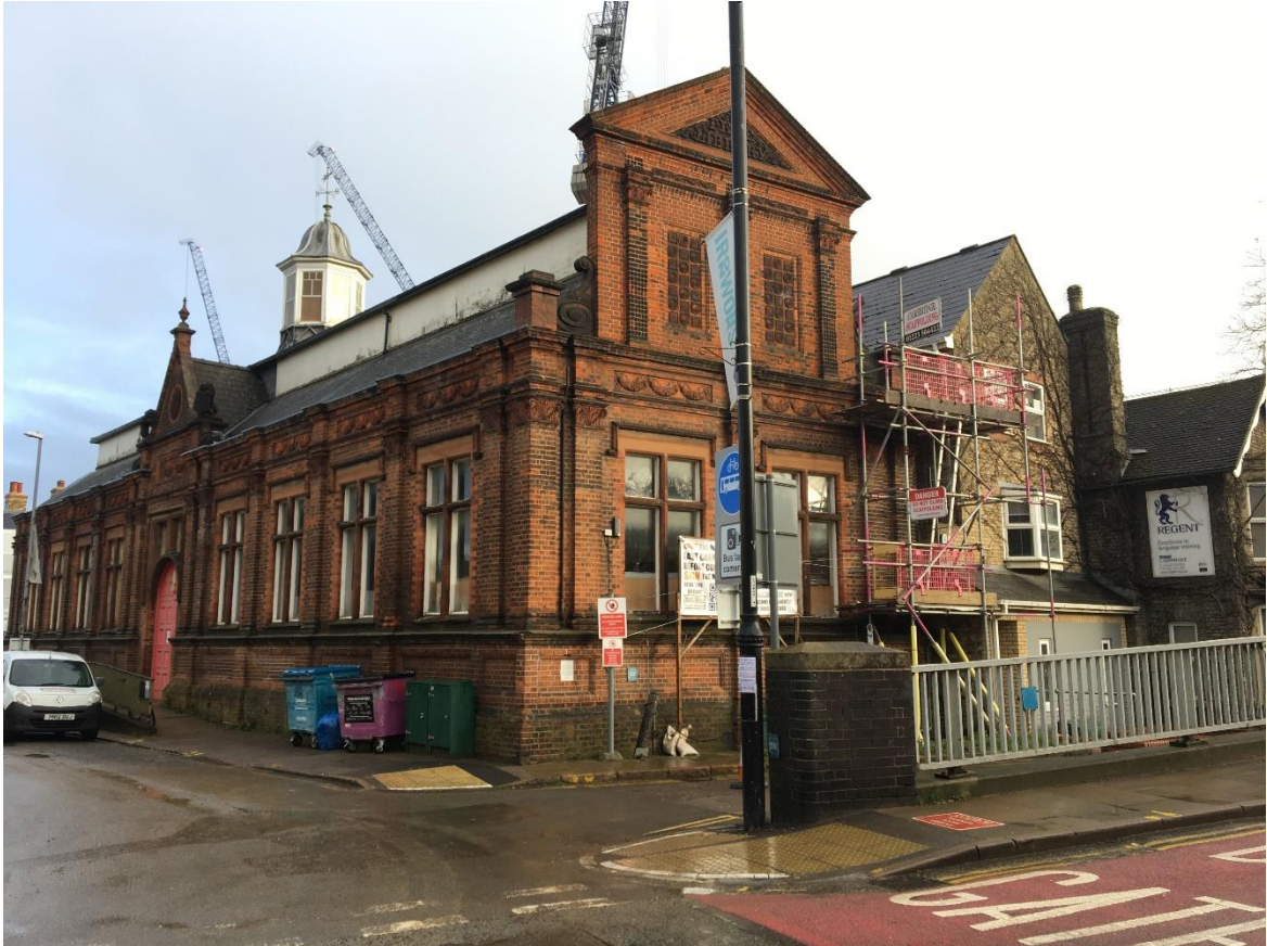
Figure 12 View of the Cambridge Branch Library from Mill Road
