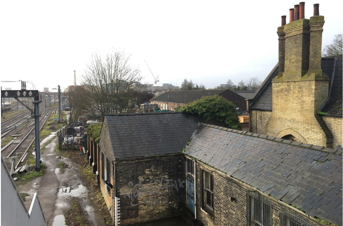
Figure 15 View toward the site from the Mill Road railway bridge
