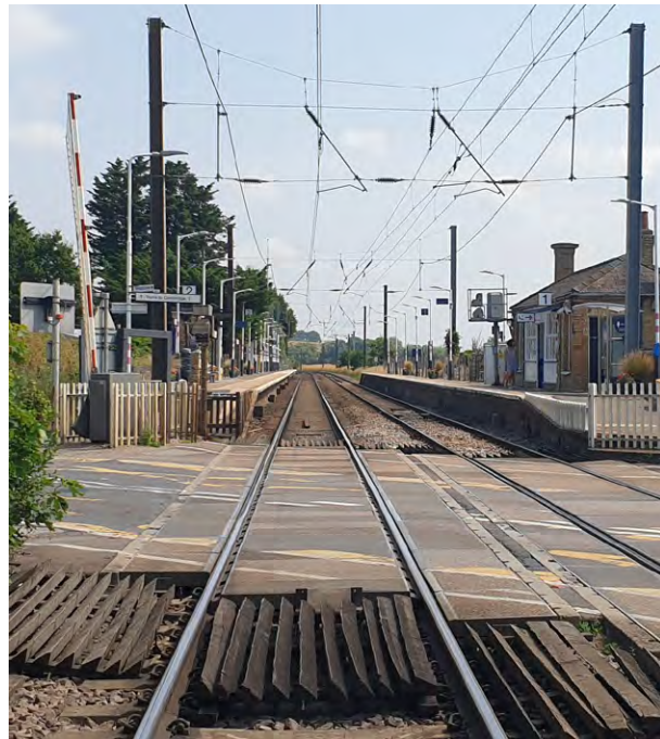
A10 Foxton level crossing
