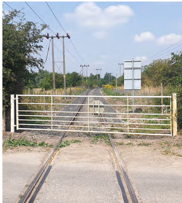
Foxton Road level crossing
