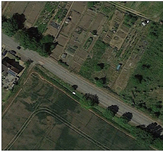
NORTH SOUTH AERIAL VIEW
