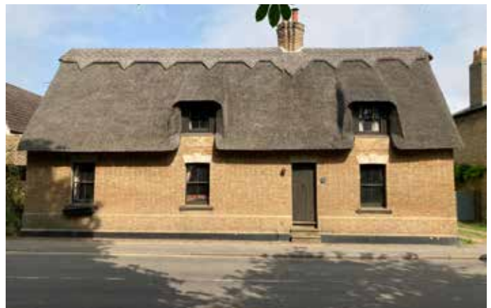
Grade II Listed - 332, High Street
