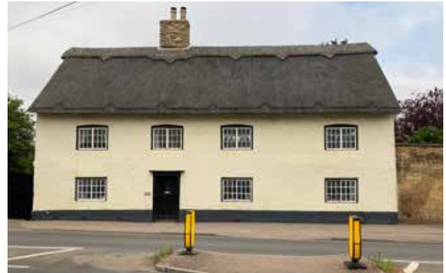
Painted brickwork is also found on a number of buildings within the village.
