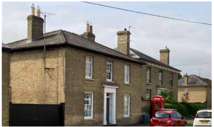
Chimneys are a prominent architectural feature to both the street and roofscape of the village.
