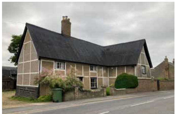
Grade II Listed - 279, High Street
