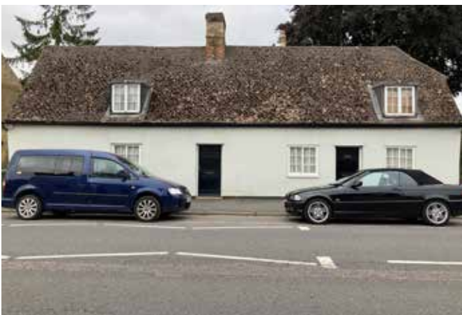
Grade II Listed - 226 & 228, High Street
