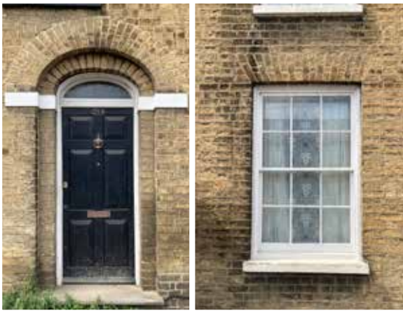
Brick detailing over doors and timber sash windows is a common architectural features found in the village on both larger villa properties and former worker cottages.
