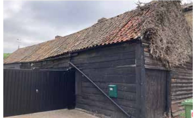
Examples can be found around the village of the original agricultural buildings in timber weatherboarding. Some have clay tiles as in this example or metal corrugated roofs.
