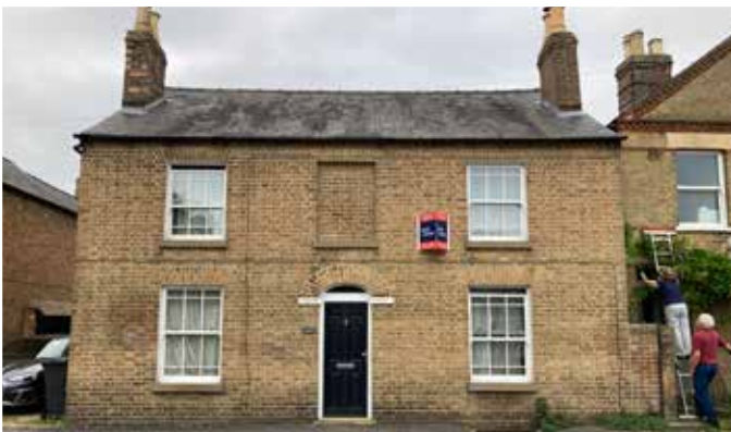
The local buff brick with a slate roof covering is the predominant material found on buildings within the village.
