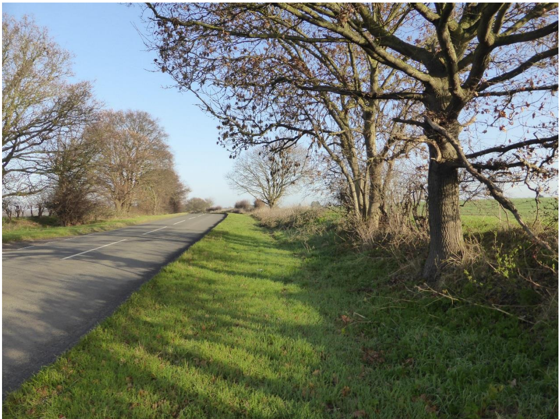
Figure 22 - Looking north. Room for verge path
